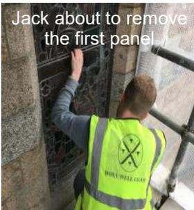
For the next few days you could hear the chip, chipping sound of the masonry being painstakingly removed from both inside and out in order to remove the panels. Work progressed well and by the end of Wednesday the whole window had been removed and secured in the van, ready for Jack to return on the Friday boat.
